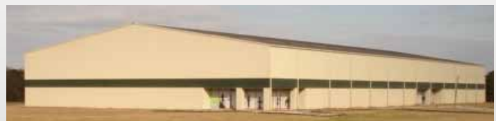
Prattville, AL plant – Opened 2007
